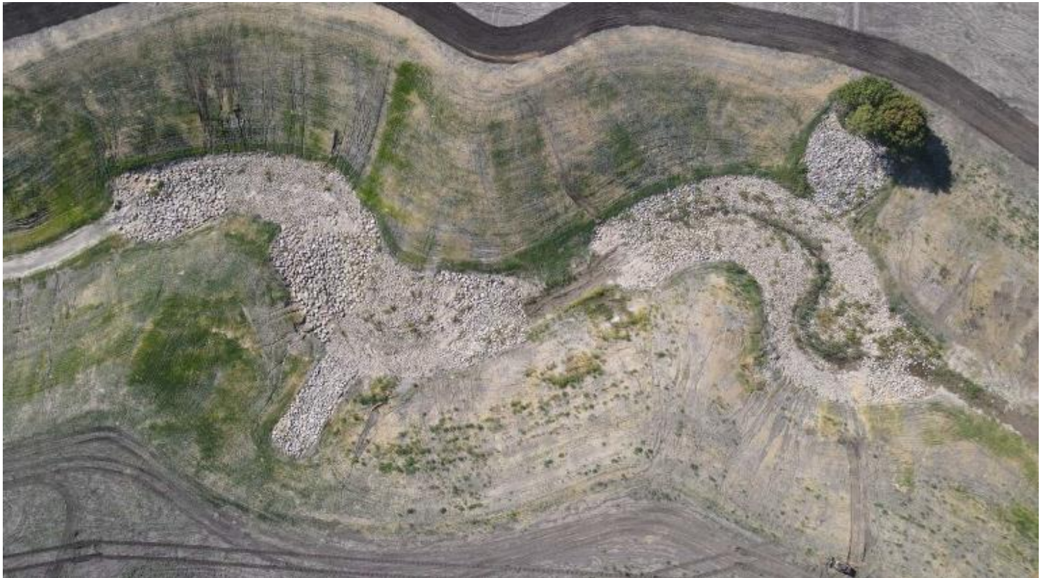
Lake Traverse Water Quality Improvement Project No. 1 Phase 3 from above
